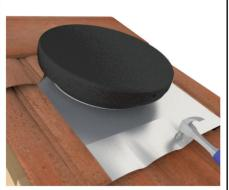
Gently form the bottom and side edges of soaker tray to profile of the tiles.
